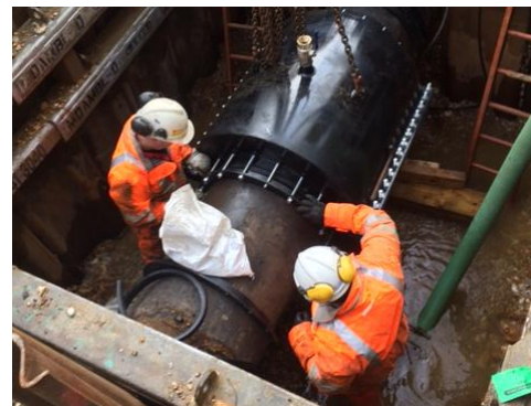
First End Ring Installed
