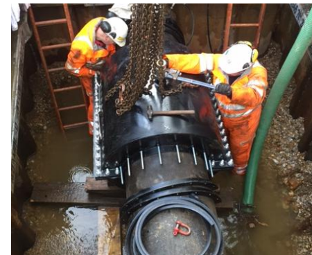
Installation of new clamp under-way – top & bottom shells in place
