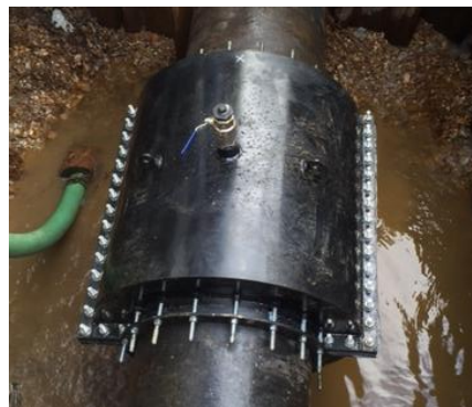
Final plug tested, valve in off position, repair complete
