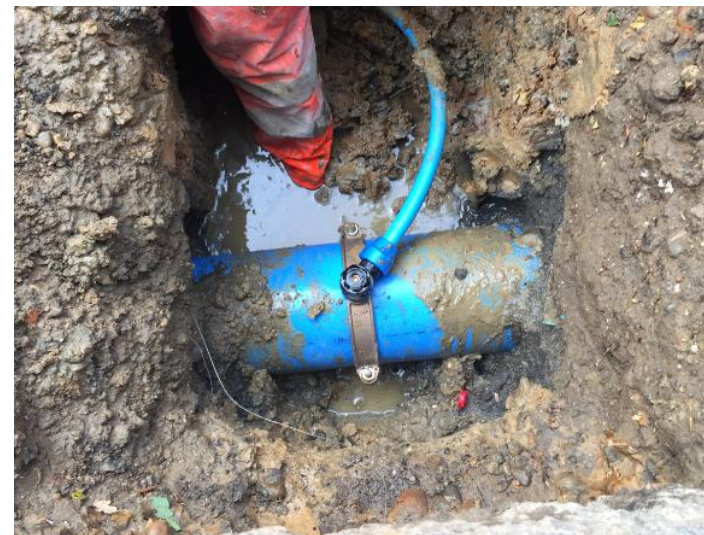
Service now re attached to the new main using a short piece of PE service pipe to divert it from the old black PE service. Complete at 9:44.
