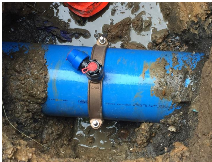
Ferrule strap installed onto a live 200mm MOPVC Main at Great Horkesley Near Colchester – started at 9:31.
