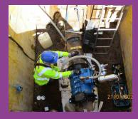
3. EM (end milling) machine in place making slot across the pipe.
