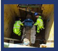
2. Valve body mounted on pipe.
