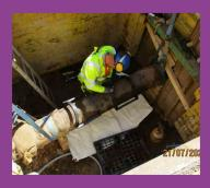
Pipe cleaned and taped, ready for install.
