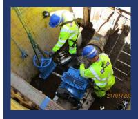
4. EM (end milling) machine removed and bonnet ready to be mounted.
